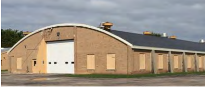
Osborn Avenue Garage:
